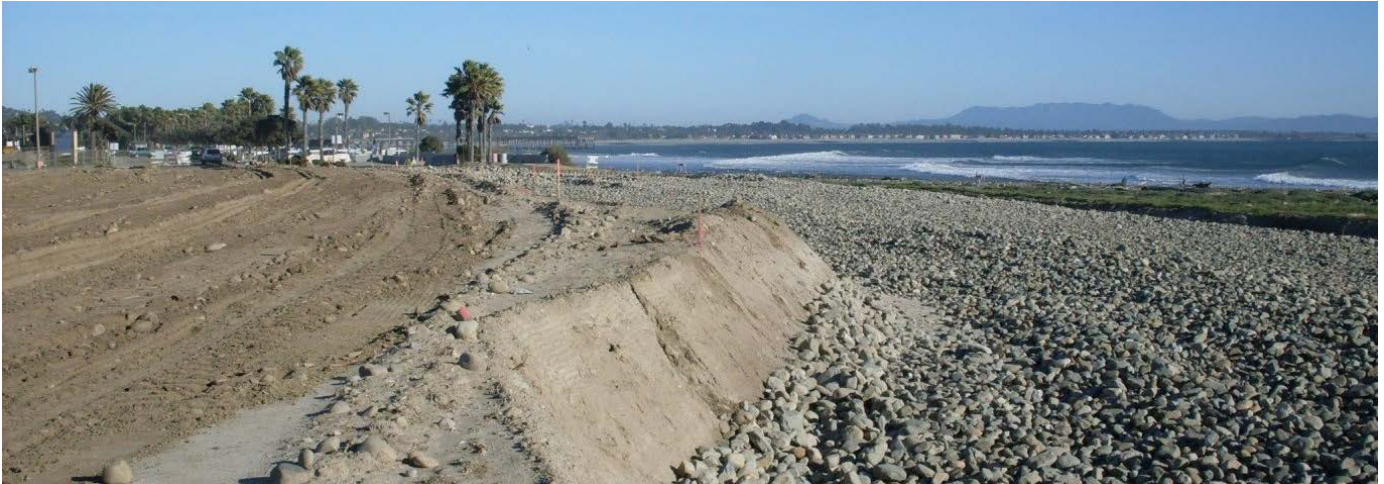
▲ Figure 13: After the eroded parking lot and bike path were excavated, cobble was imported and covered with sand to restore the cobble beach. 2011. Photo credit: City of Ventura.
