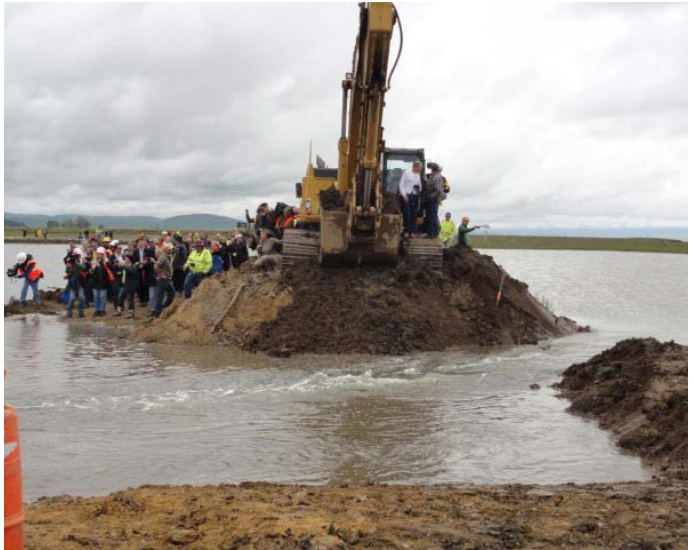
▲ Figure 32: Bayward levee was breached to restore site to full tidal action on April 25, 2014. Photo credit: USACE.
