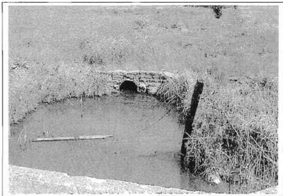
Photograph 3. Concrete culvert, camera facing southwest, April 8, 2002
