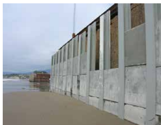
Installation of new caisson walls in 2011 substantially improved the structural integrity of the seaward-facing side of Pier 421-2.
