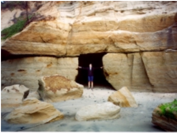
Sea cave, note rocks in foreground from past bluff failure.
