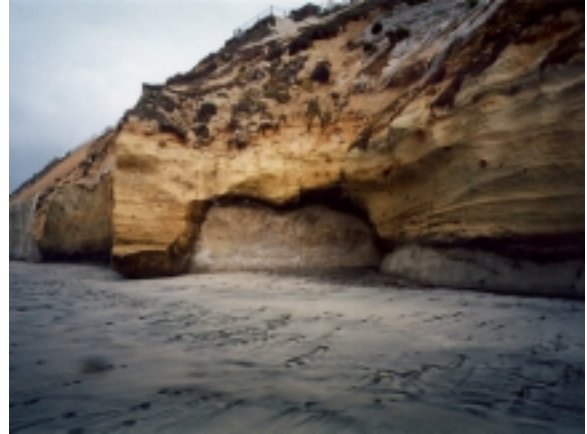
Typical sea cave fill. Note minimal encroachment onto beach.
