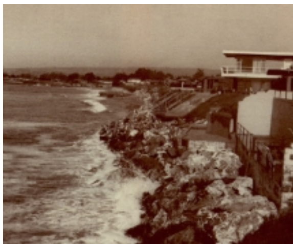
Example of rock revetment used as shore protection device. Source: Shore Protection in California.
