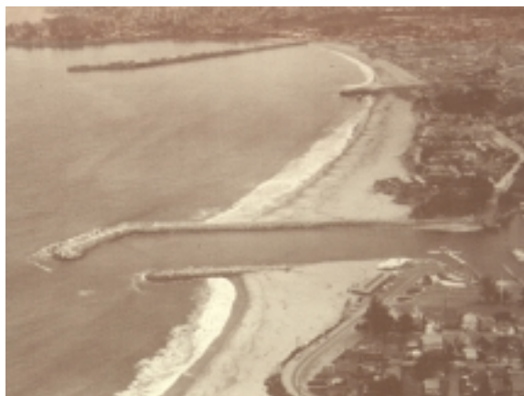
Example of rock jetties protecting a harbor entrance. Source: Shore Protection in California.
