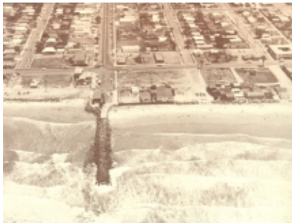
Rock groin used to limit sand movement along the shore. An effective shore protection device if sand fill is made on the up coast side. Source: Shore Protection in California.
