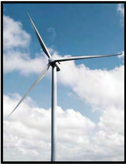
Figure 4.3.1. Turbina Sapiens (SWT-6.0-154) by Siemens
