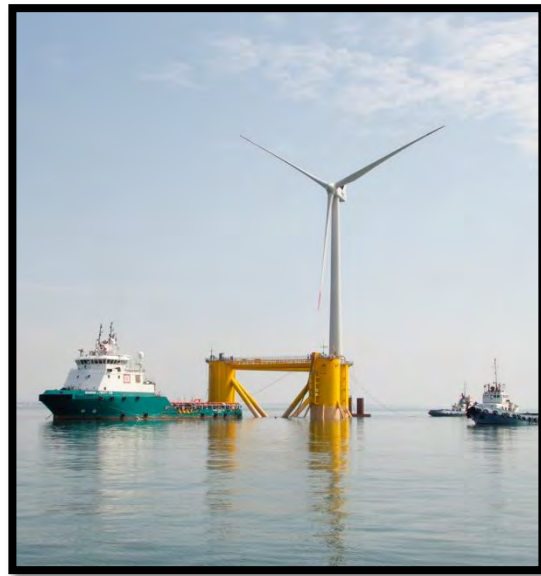
Figure 4.3.2. V80-2 MW Gridstreamer Turbine by Vestas with WindFloat Foundation Technology by Principle Power
