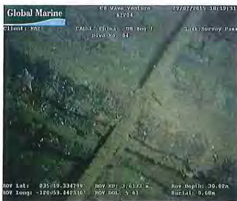
Cable suspended over rock KP3.613
