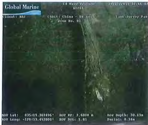
Cable damage on rock outcrop KP3.679
