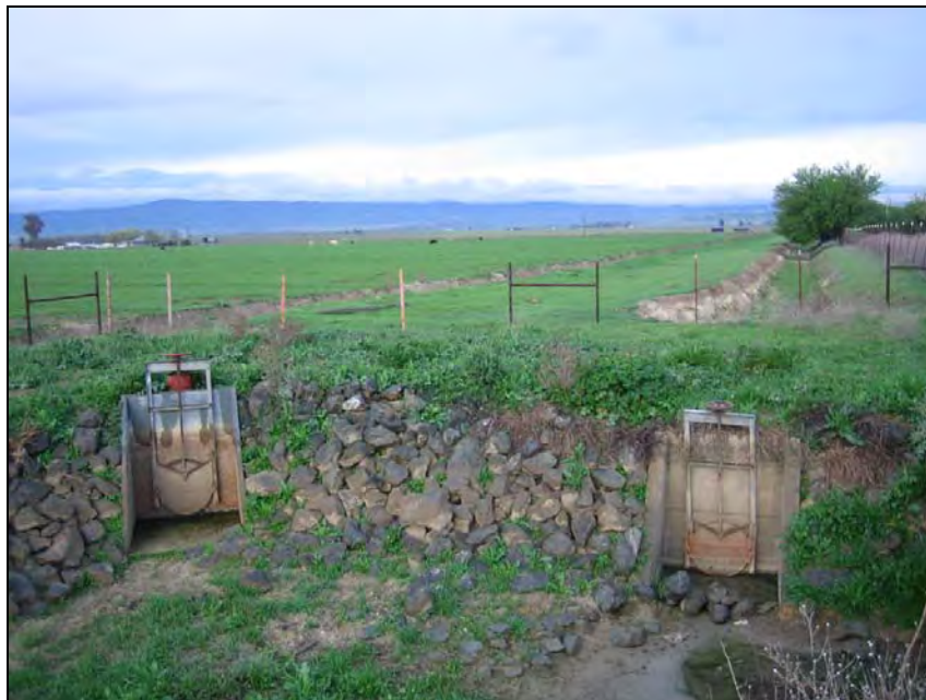
Southwestern overview of two ditch gates opening into two parallel spurs off the Goodnow Slough; 03/20/2007; IMG_1389.
