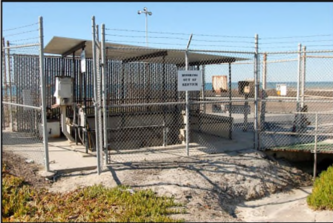
BEACH VALVE PIT EXTERIOR
