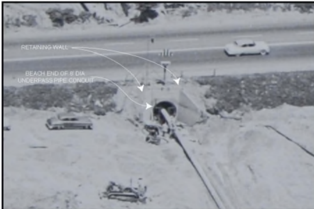
Photograph of original construction in 1953. The termination of the underpass pipe conduit (8' dia) and retaining wall (wing walls) can be seen. The underpass end structure is shown under construction. The retaining wall is now located underneath the #2 southbound lane of Carlsbad Blvd. The end structure, when constructed, extended another 16'-7-1/4" toward the beach.
