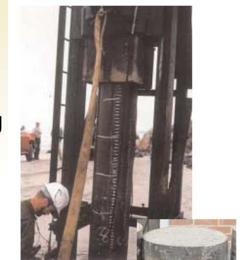
Performing pile driving analysis (PDA)
