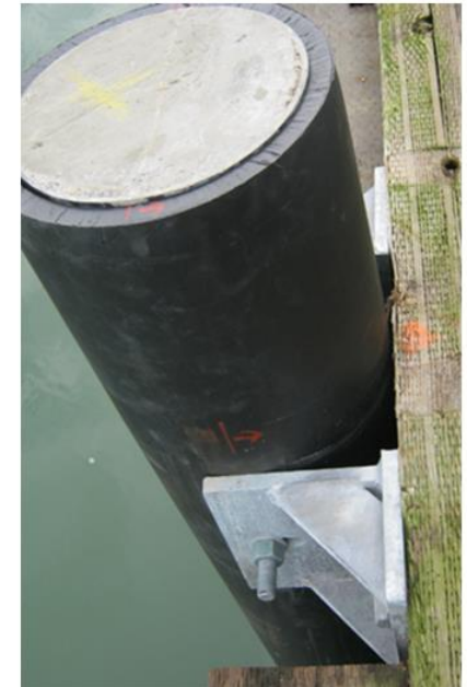
Berth 9/11 - Composite piles with timber waler system, and new concrete curb.
