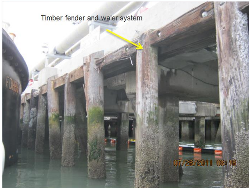
Main Wharf, Berth 9 (before) Approach velocity limitations, requiring AAS velocity monitoring.
