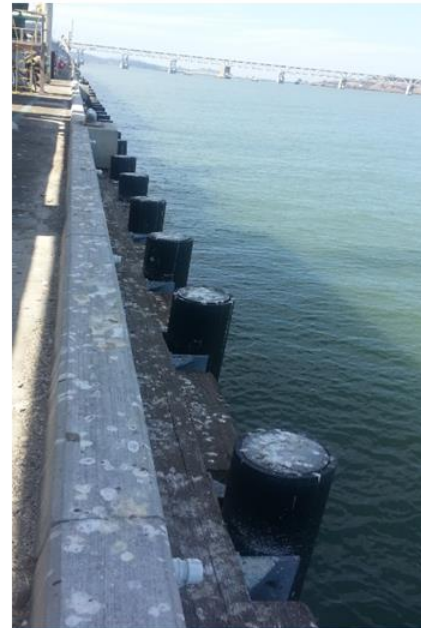
Berth 9/11 - Composite piles with timber waler system, and new concrete curb.
