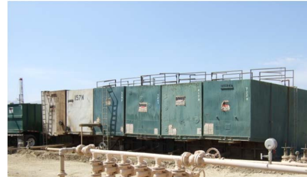
Temporary 500 bbl Injection Water Tanks
