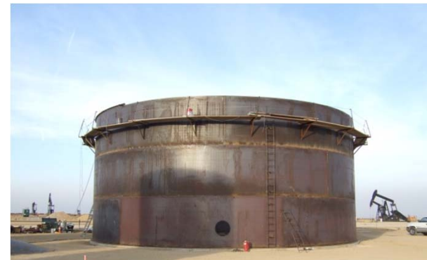
New 10,000 bbl Injection Water Tank
