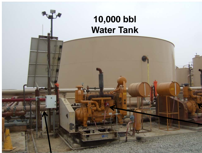
Main Panel with SunWize 24VDC Solar Array
