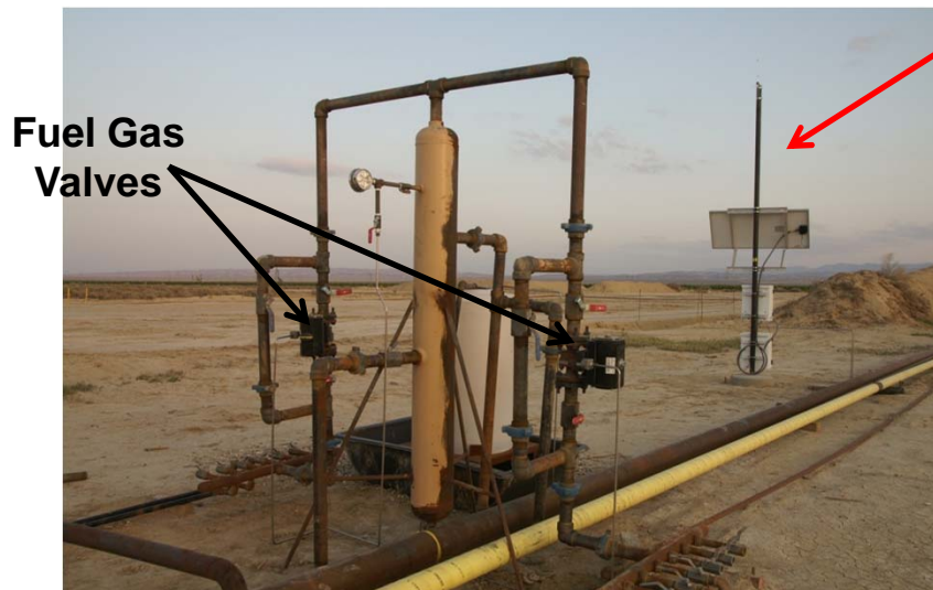
Remote Panel behind Fuel Gas Shutdown Station
