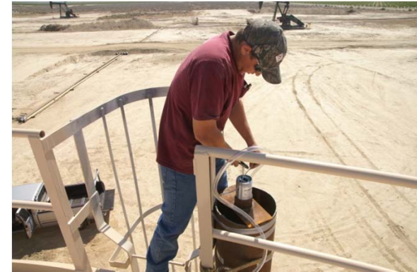
Wiring the Ultrasonic Level Transmitter for Calibration
