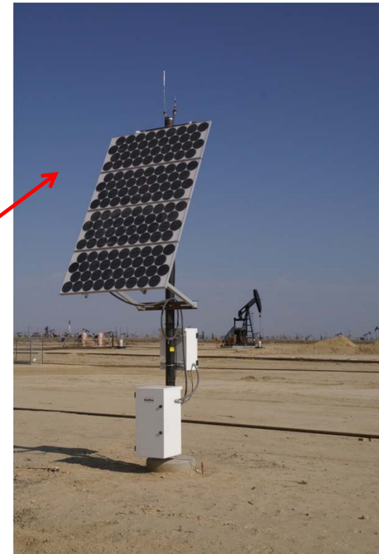
Main Panel with SunWize 24VDC Solar Array
