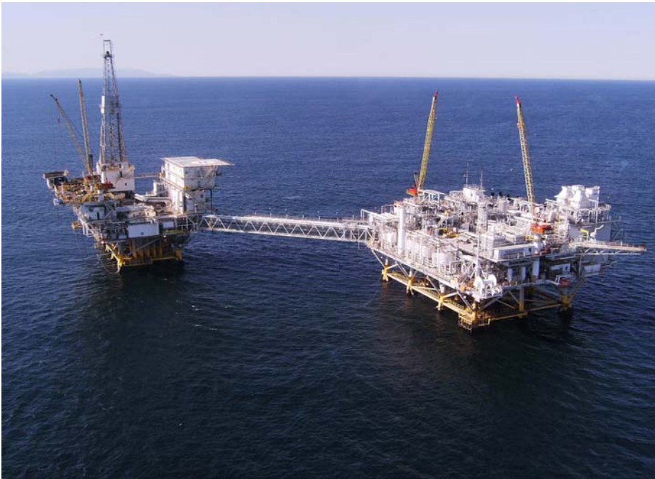
Platform Ellen 80 Well Slots 17 Empty
