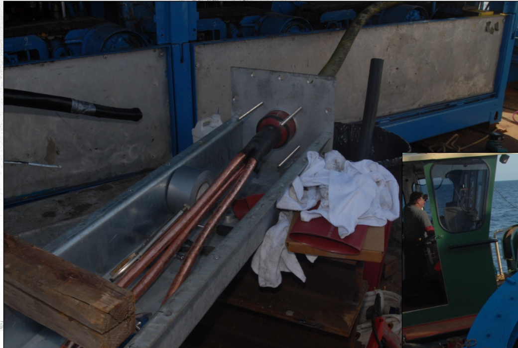
Cable splice under construction.
