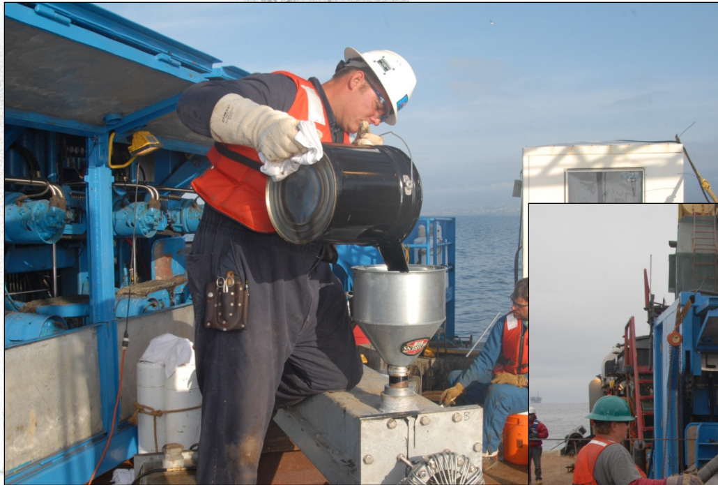
Splice box being filled with No-Void.
