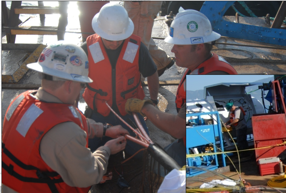
Hampton Tedder crews preparing cable end for testing.
