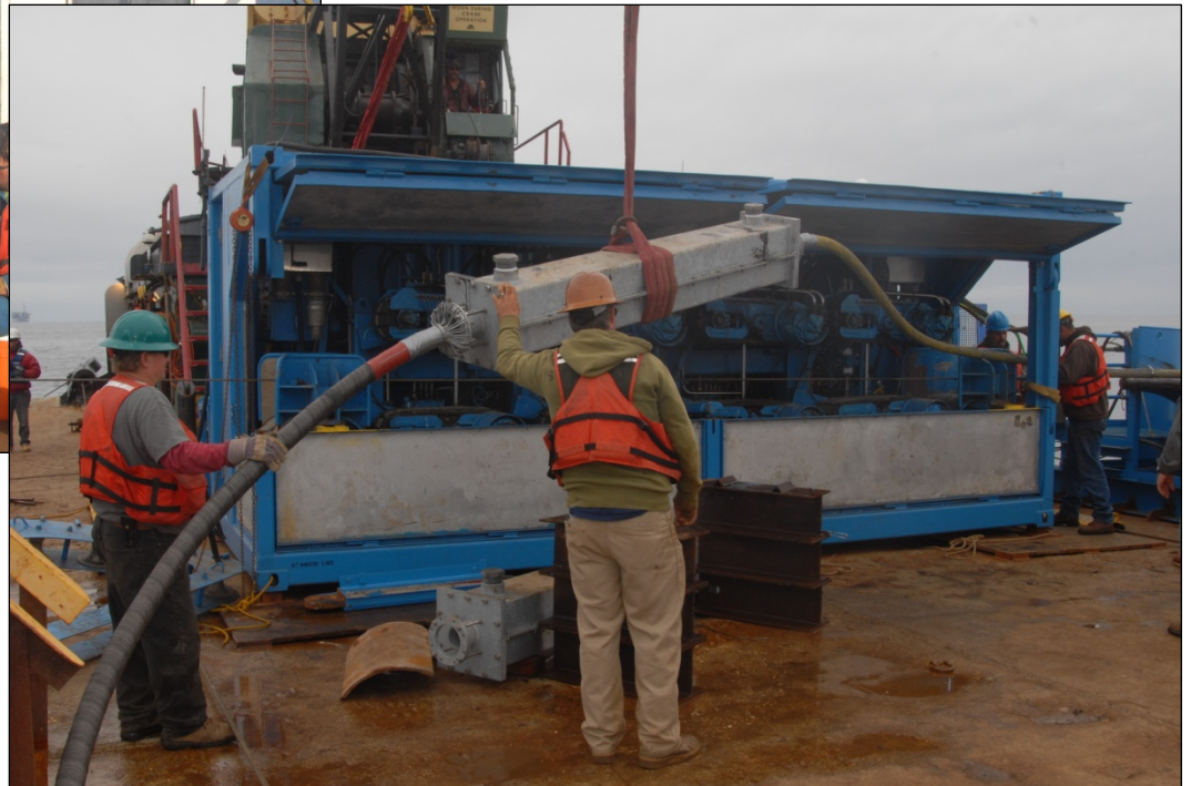
Splice box rigged and ready to overboard.
