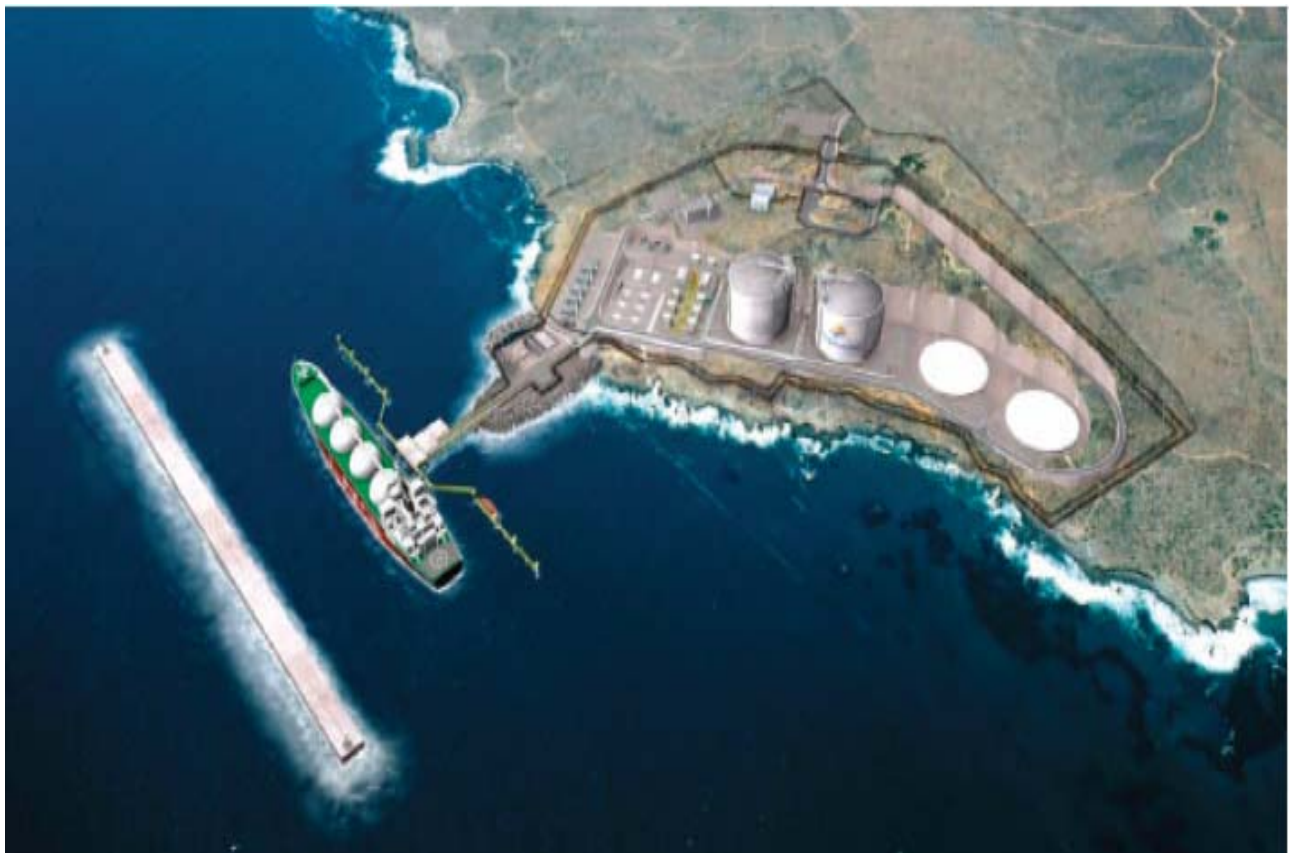
Figure 1: Typical nearshore facility. This one is being constructed at Costa Azul, Mexico.
