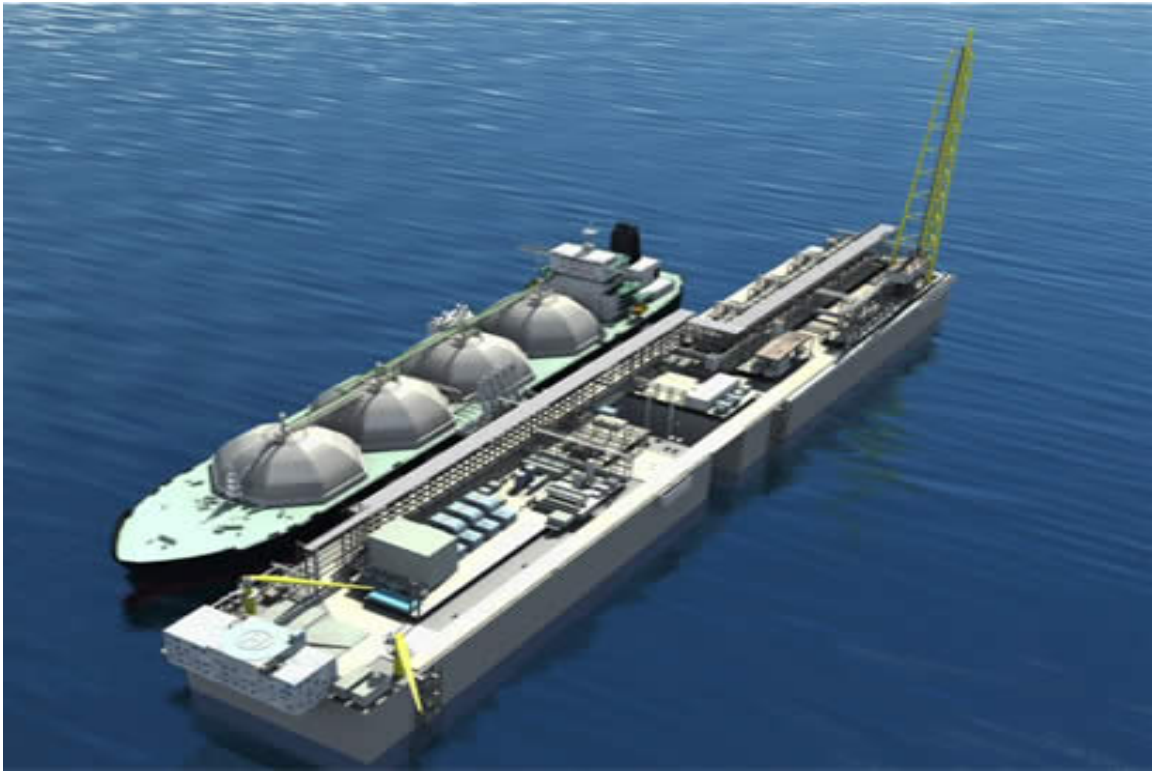
Figure 5: Example of Gravity Based Structure (GBS) with tanker moored next to it.
