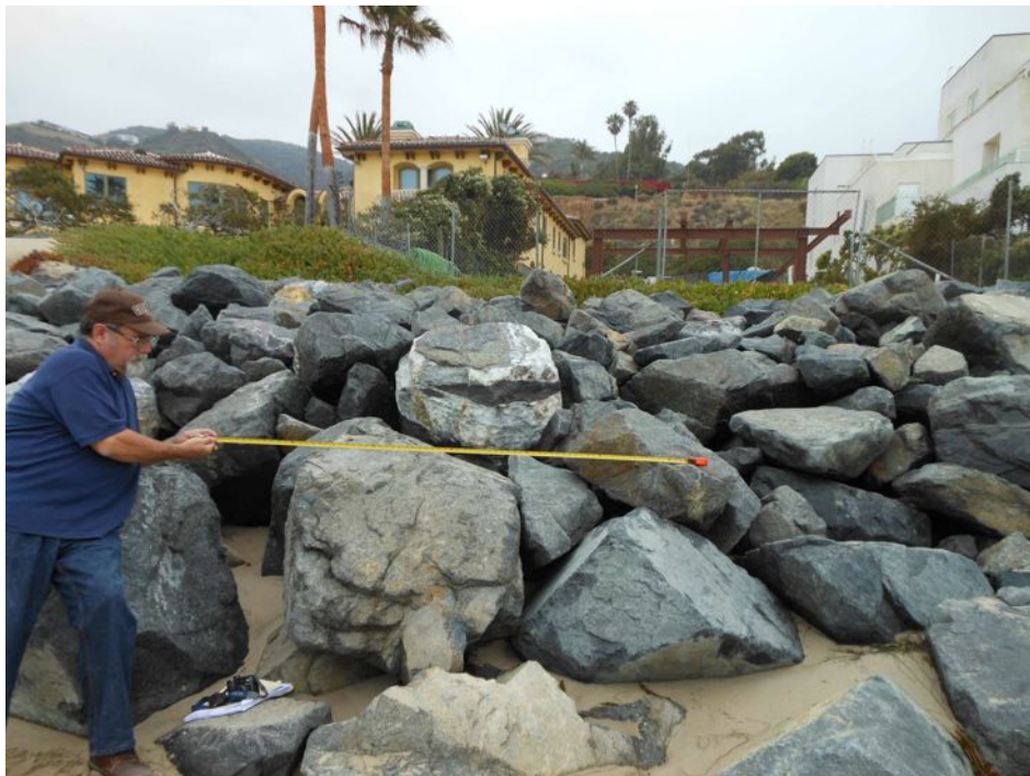
Photo 4B. In the middle wall section, this view near 31038 Broad Beach, shows the rock diameter to range from 1-ft to 3.5-ft in diameter. Wall height is approximately 6-ft high.
