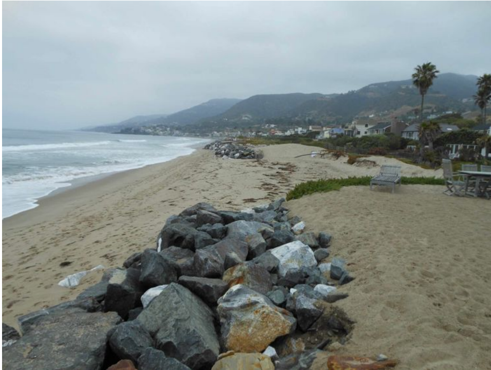
Photo 5B. An approximate 200-ft long gap in the revetment wall, located near 30822 Broad Beach Rd., was created at the time of placement. Wall in this area is approximately 6-ft high
