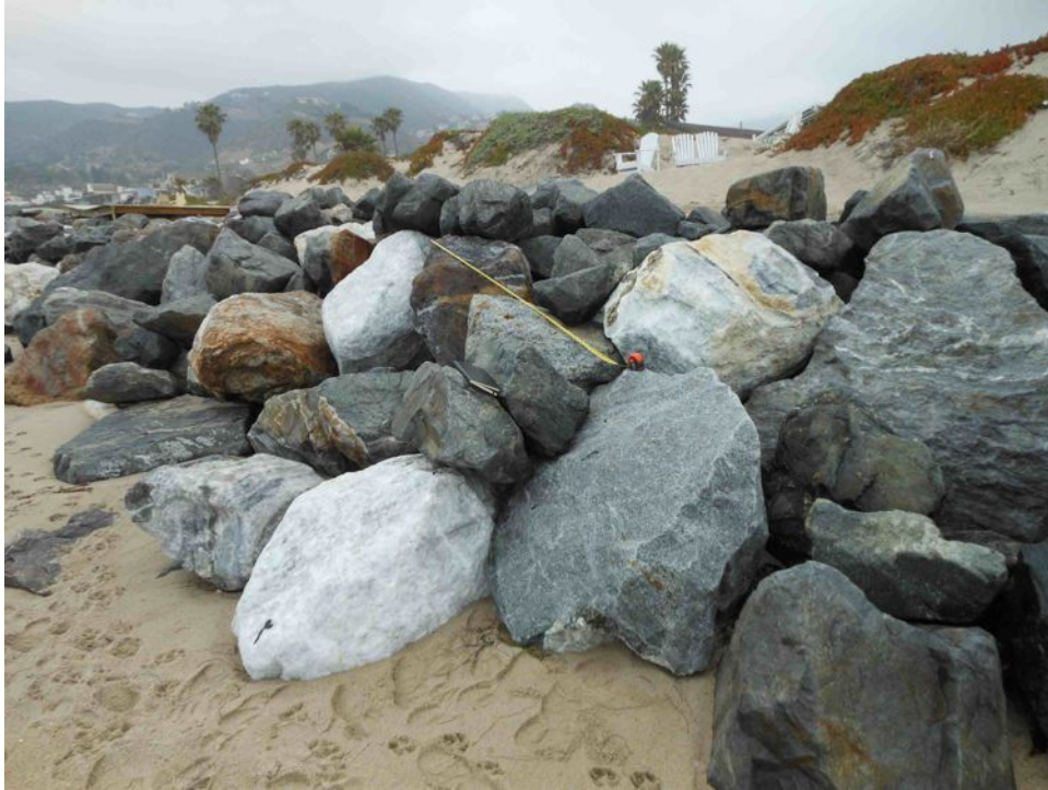
Photo 5A. Height of rock revetment wall at east end of wall, near 31078 Broad Beach Rd, is approximately 6-ft high. Measuring tape is 6-ft long. Rock size in this area ranges from 1-ft to 3.5-ft in diameter.
