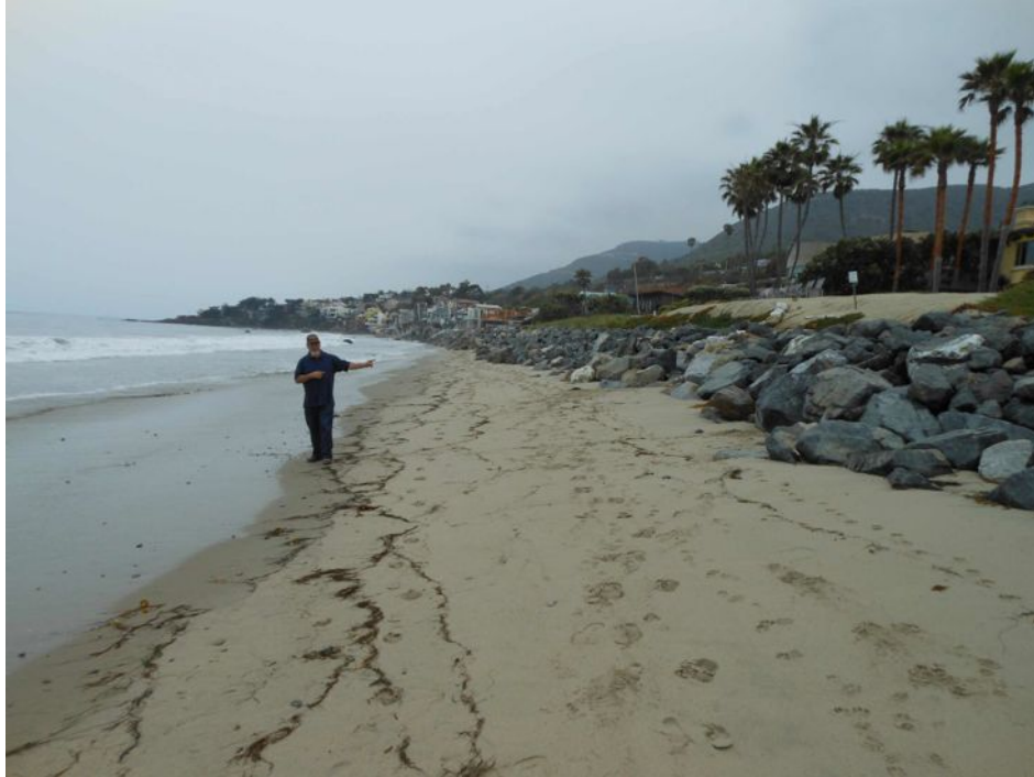
Photo 4A. In the middle section, the height of the wall ranges from 6-ft to 8-ft high. For the most part the rock sizes appear to be adequately stable for the wave attacks during the last 2 years as few rock pieces were displaced.
