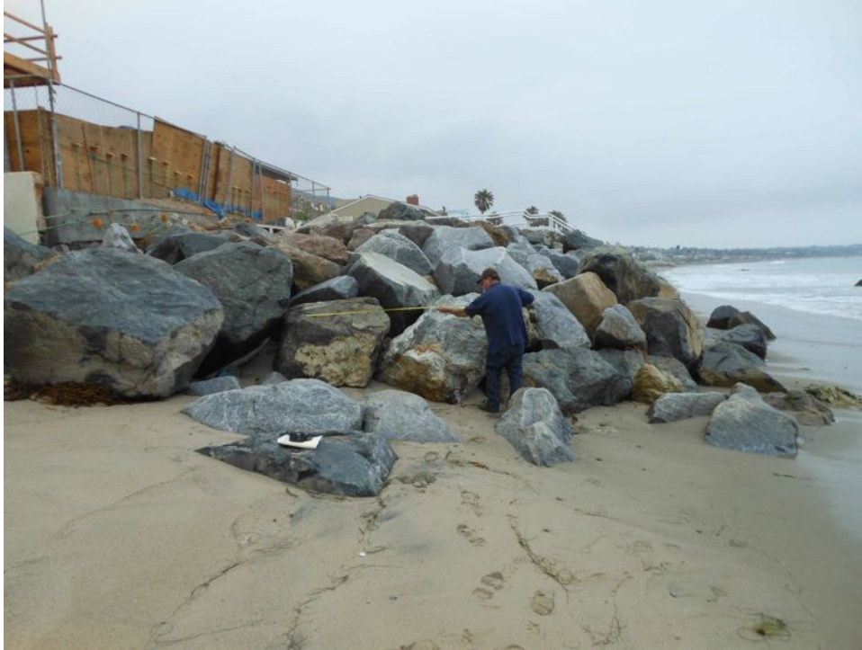
Photo 3A. Size of exterior rock revetment at west end of wall, near 31346 Broad Beach Rd, ranges from 4-ft to 6-ft diameter. Measuring tape extends about 5-ft left of the person's hand. Rock is plutonic igneous and gneiss rock type.
