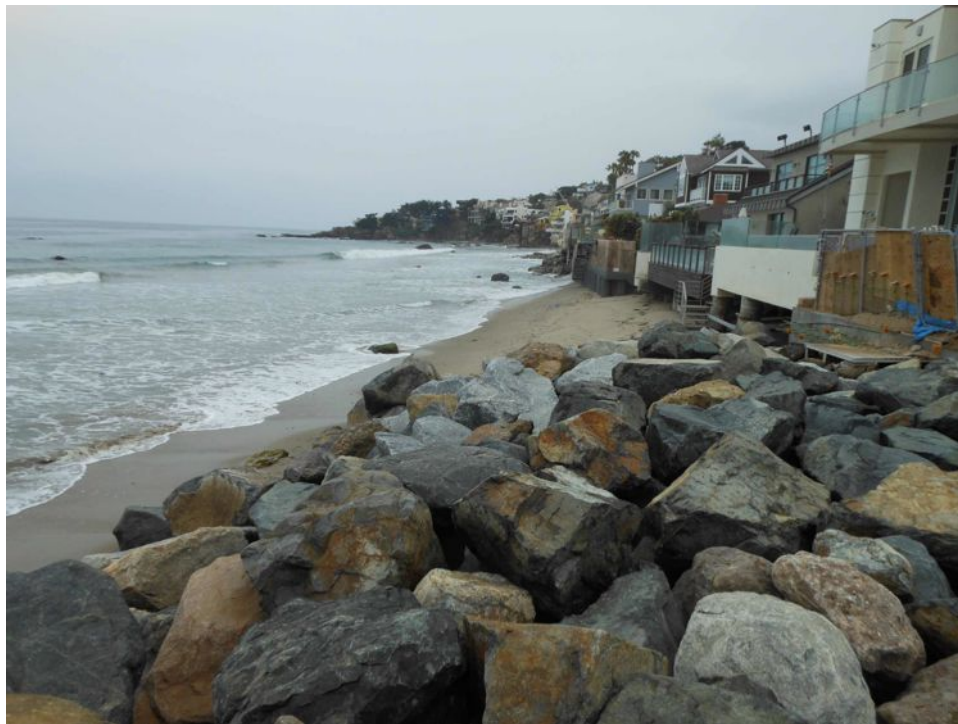
Photo 3B. An approximate 200-ft long gap in the revetment wall was created at the west end, west of 31346 Broad Beach Rd; photo taken from western beach access. Wall height in this area is approximately 10-ft to 12-ft. Note that erosion has exposed the substructure support of these residences.
