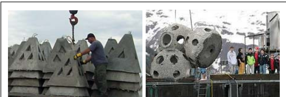
The artificial reef at Smitty's Cove used pyramid shaped fish havens (left) and reef balls (right). Monitoring has demonstrated that the artificial reef structures have a marine community make up that is similar to nearby natural reefs (e.g., Bush Banks Pinnacle).
