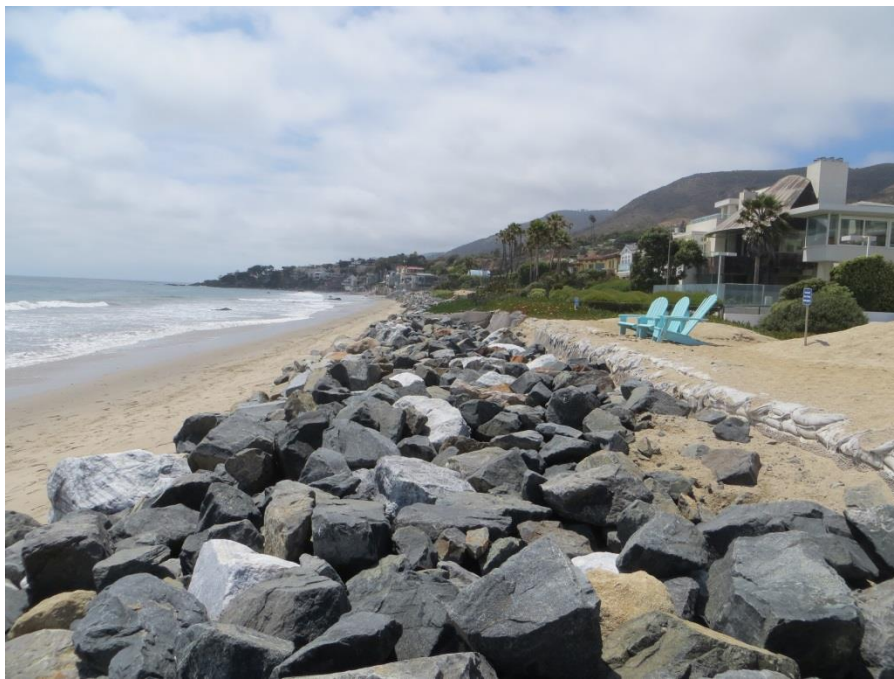
Figure 9. Images showing the location of the 2010 emergency rock revetment against the pre-revetment sandbags and other shoreline stabilization materials.
