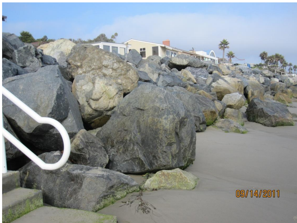
Figure 2-4. Revetment at the east end of Reach B. Notice large rock size.
