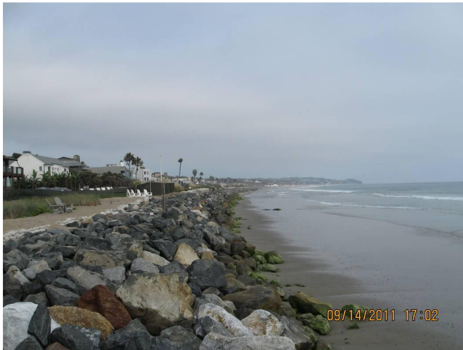
Figure 2-5. Central portion of Broad Beach and emergency revetment installed in February 2010, Reach C.
