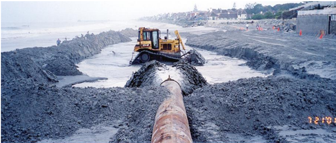
Figure 8-2. Placement of dredged sand on the beach showing the training dike.
