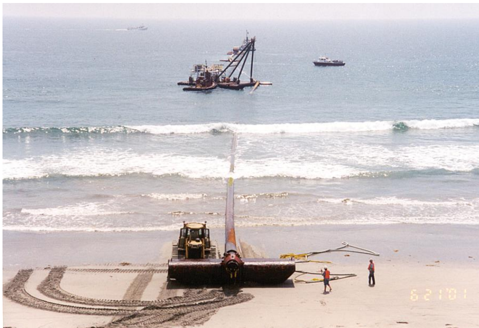
Figure 8-1. Dredge discharge line to beach.
