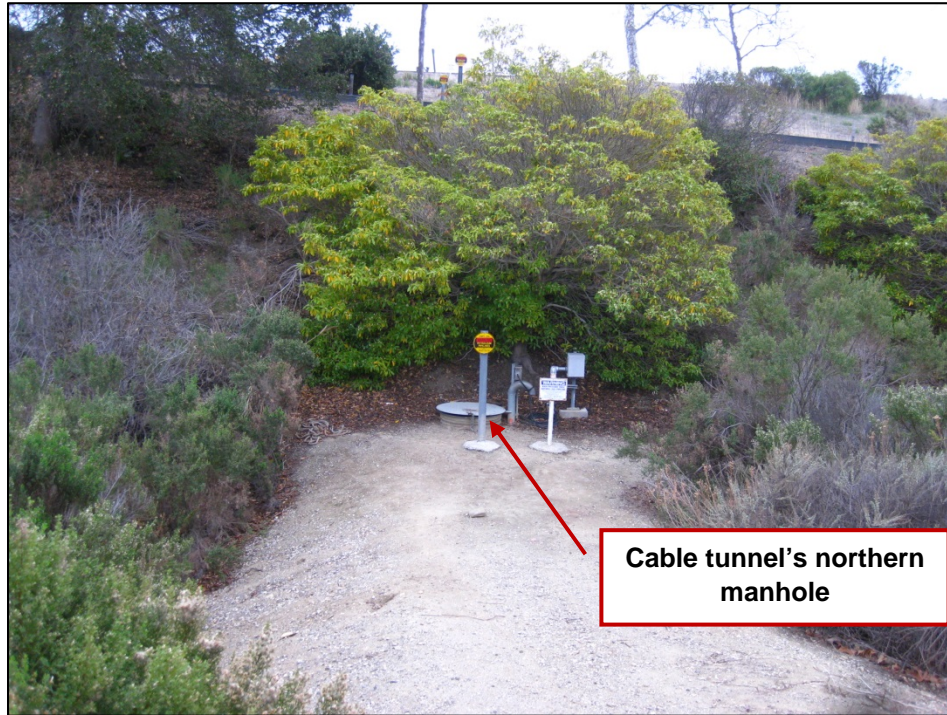
Figure 3.4-1. View of Proposed Work Area at Lower End of the LFCPF
