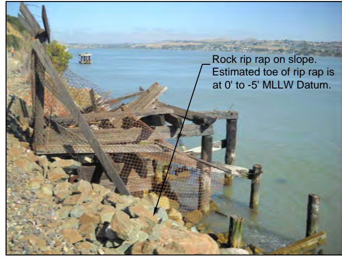
Photograph of Section H with Section J in the background
